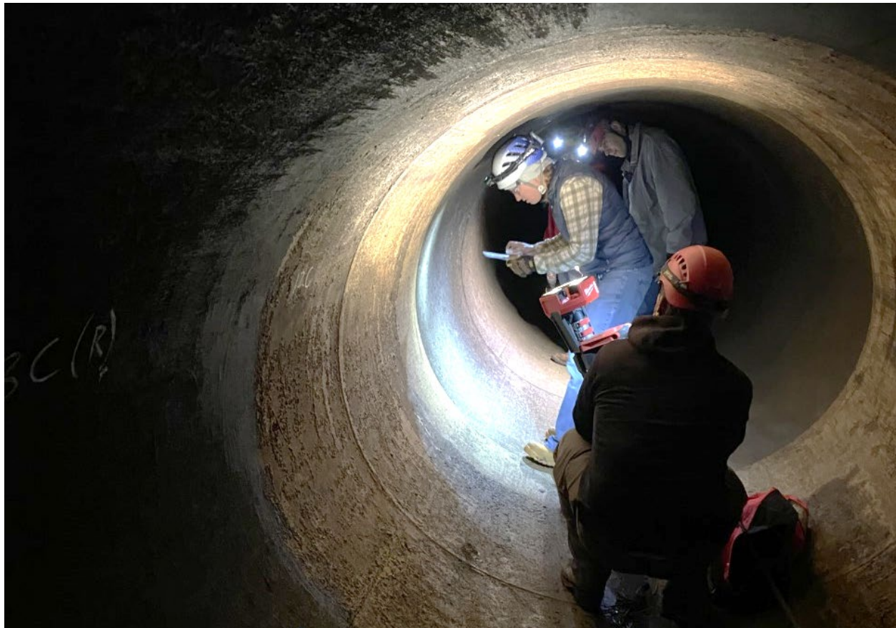
Figure 15.—Beta testing of the Survey123 tool during a siphon pipe interior coating inspection.
